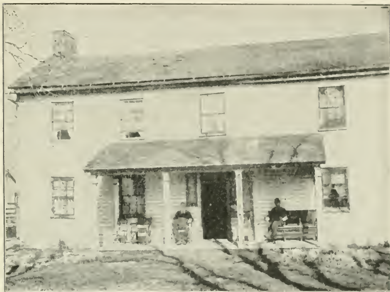
HOME BUILT BY DAVID TAYLOR 1825-6. PROPERTY OF EDWARD LIVINGSTON TAYLOR.
